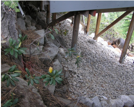
Figure 16: Armor under elevated
