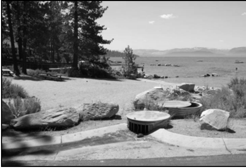
Figure 1: Downstream end of a stormwater conveyance system showing sediment traps as the last mechanical treatment before entering the Lake
