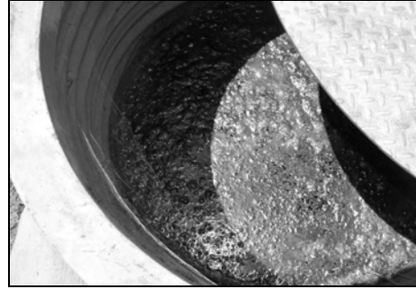
Figure 1: Downstream end of a stormwater conveyance system showing sediment traps as the last mechanical treatment before entering the Lake
